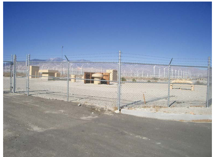
Southerly Desert Water Agency Water Well Site
