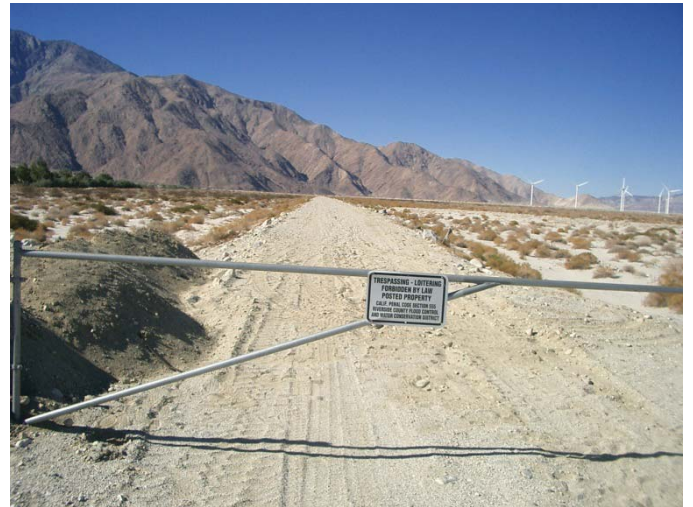
Northerly Perimeter/Whitewater River Flood Control Levee
