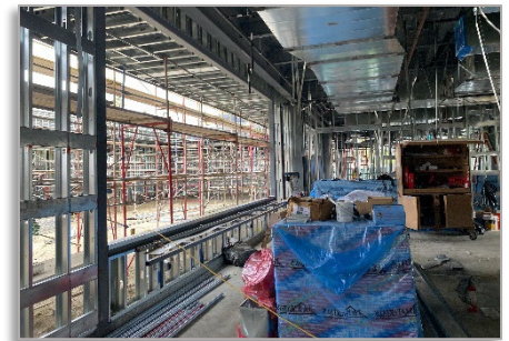
CDE Classroom Interior
