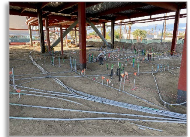
Slab on Grade Electrical
