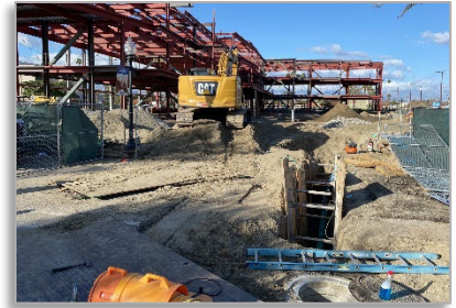
Water and Sewer Connections
