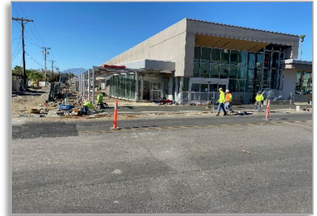
Exterior at Main Lobby
