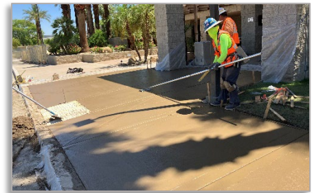
Handicap Access Ramp and Sidewalk
