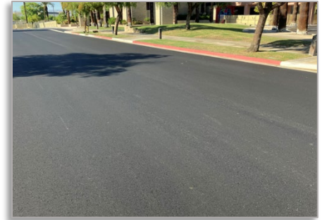
Paved West Roadway
