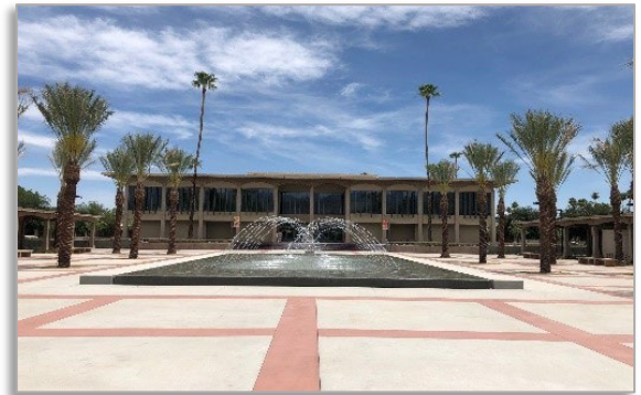
Central Campus Quad Renovation
