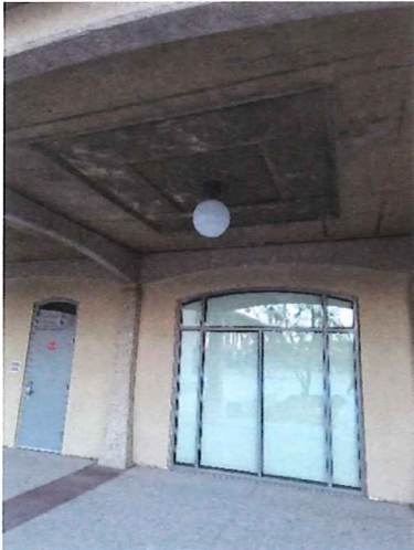
REPAIRED CONCRETE SOFFIT
