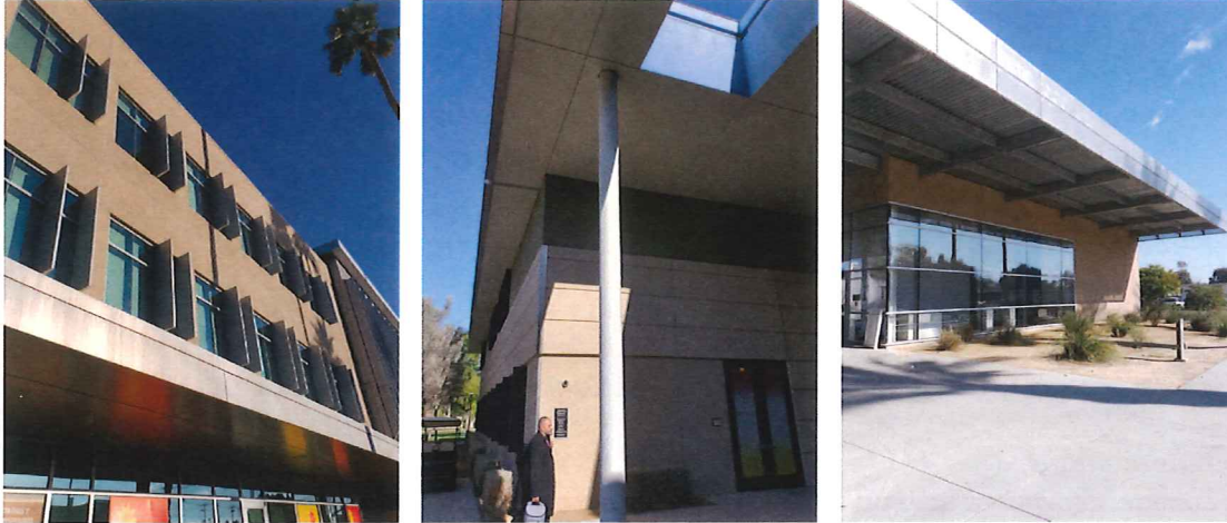
IMAGE 1.13 | SOLAR SHADING EQUIPMENT (INDIO & PALM DESERT CAMPUS)
