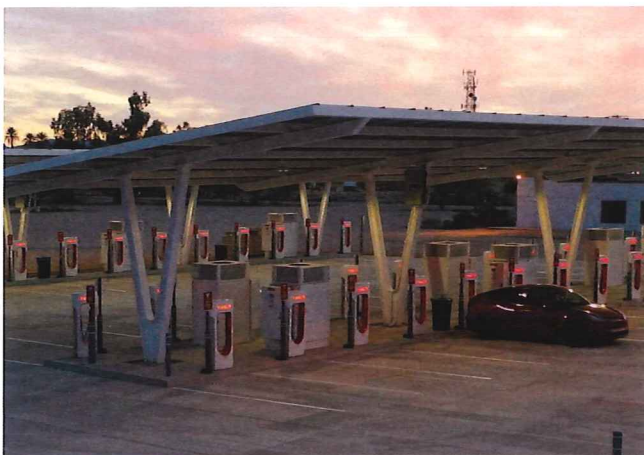
IMAGE 4.9 | STEEL FRAME PV CANOPY & EV CHARGING
