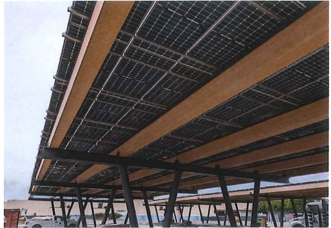
IMAGE 4.7 | SOLAR CANOPY (TIMBER AND STEEL FRAME)
