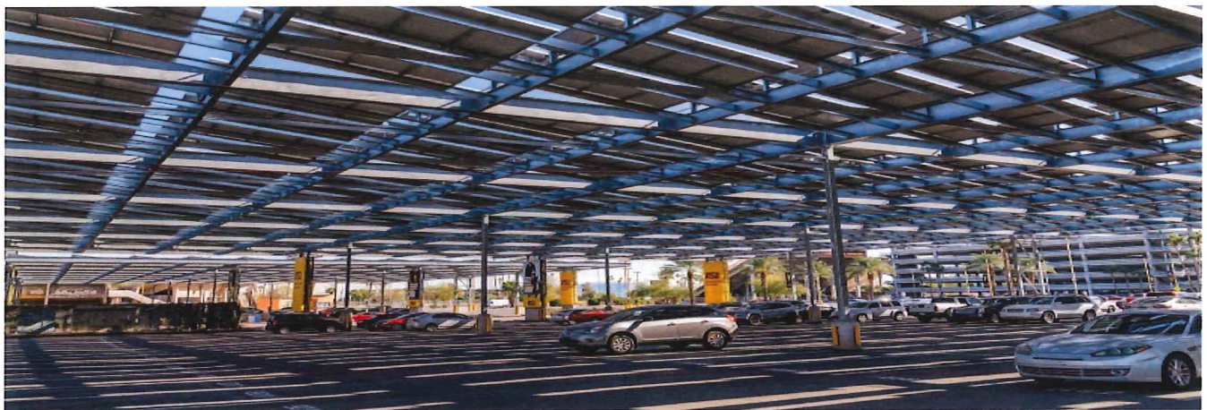
IMAGE 4.8 | CONTINUOUS MONOLITHIC SOLAR CANOPY OVER LARGE PARKING LOT, STEEL FRAMED
